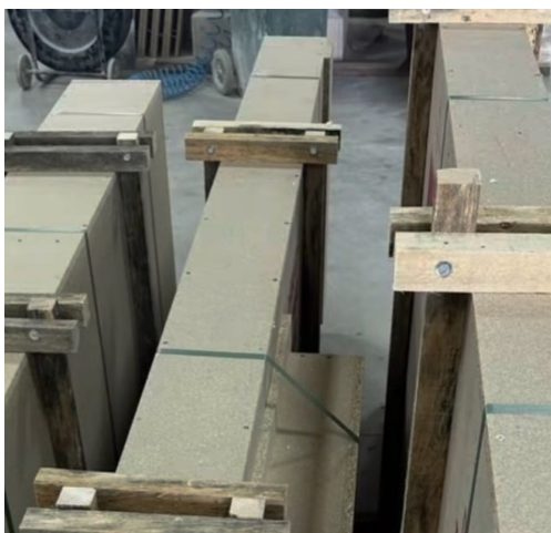
Visible removable timber clamp / post arrangement.
